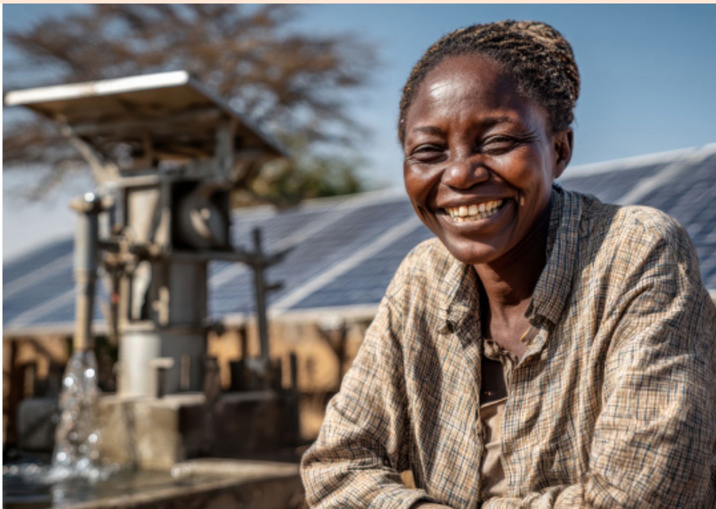
Solar Energy Water Pump
