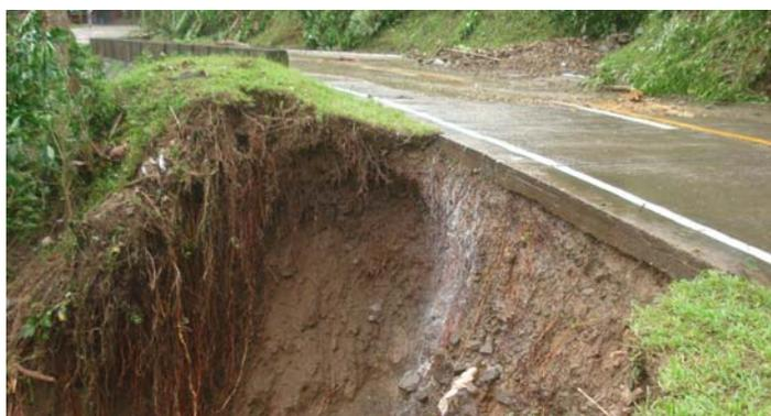
**Rainfall-induced landslide.** A portion of a road embankment slid several meters downslope due to heavy rains brought by Typhoon Frank.
